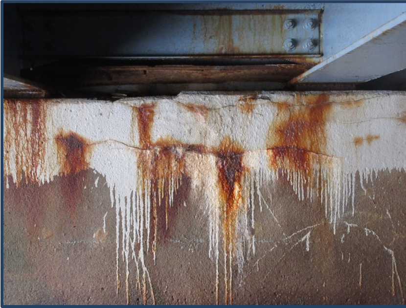
Abutment bearing seats
