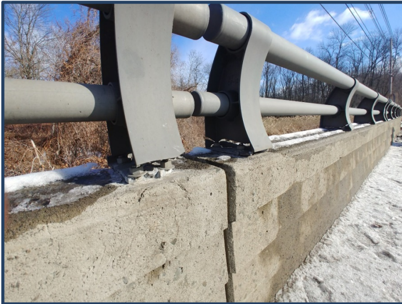
Damaged double rail element
