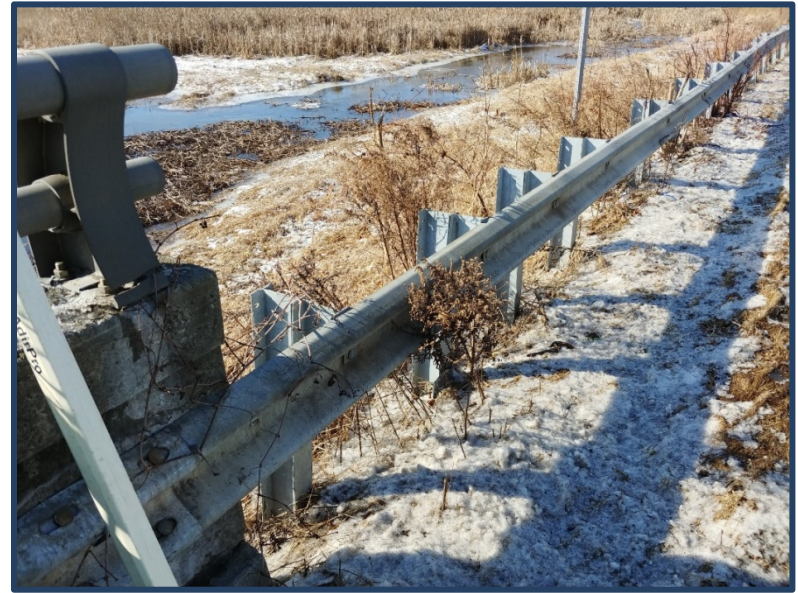
Substandard guiderail attachment
