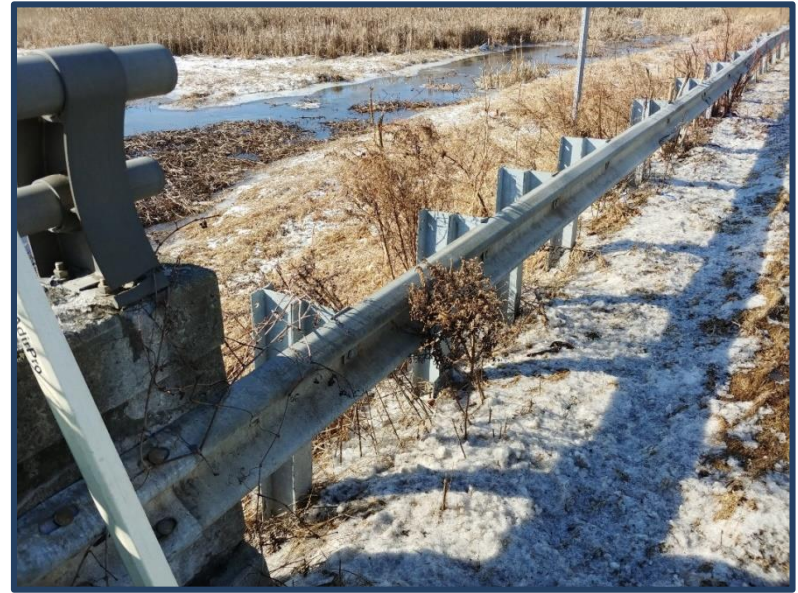
Substandard guiderail attachment
