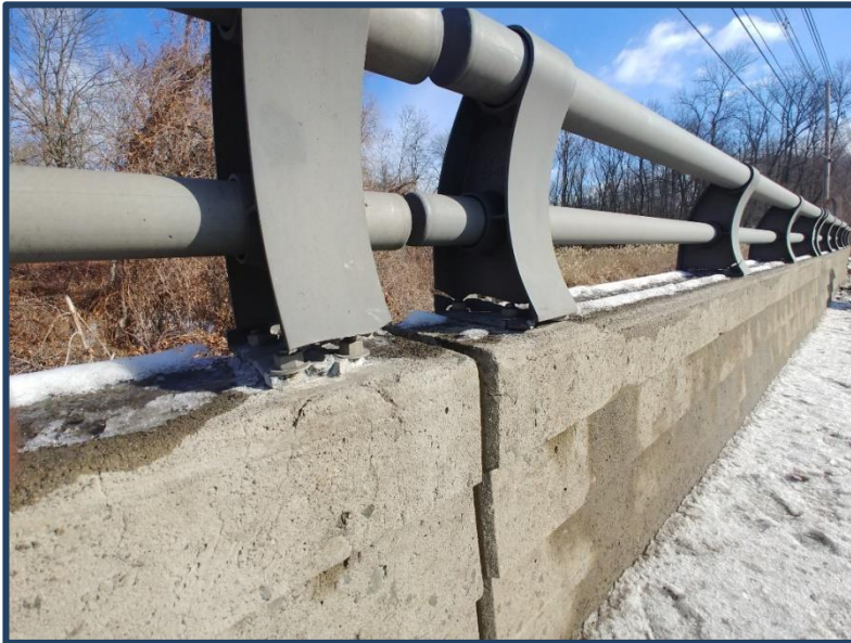
Damaged double rail element
