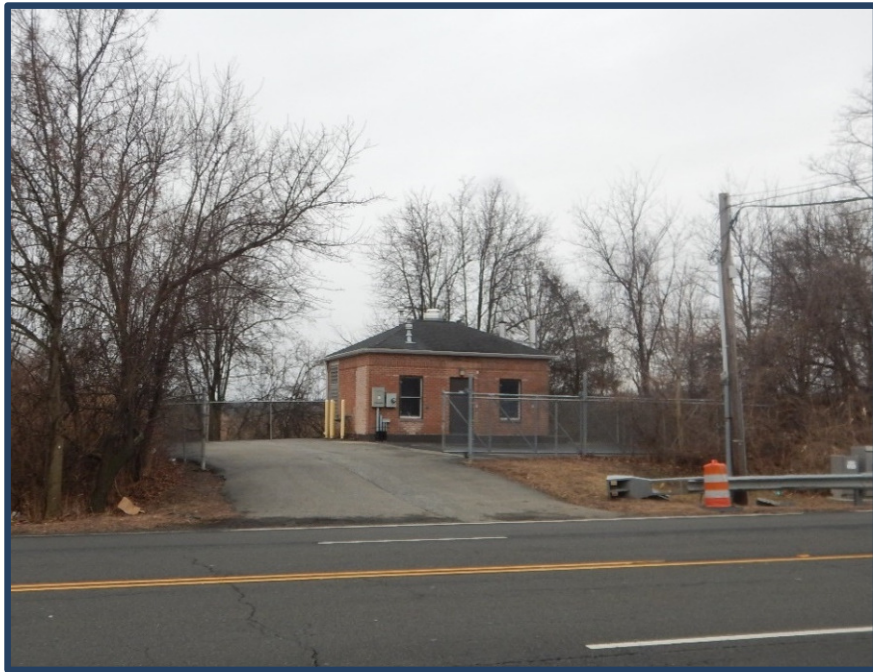
Sewer Pump Station located west of the bridge
