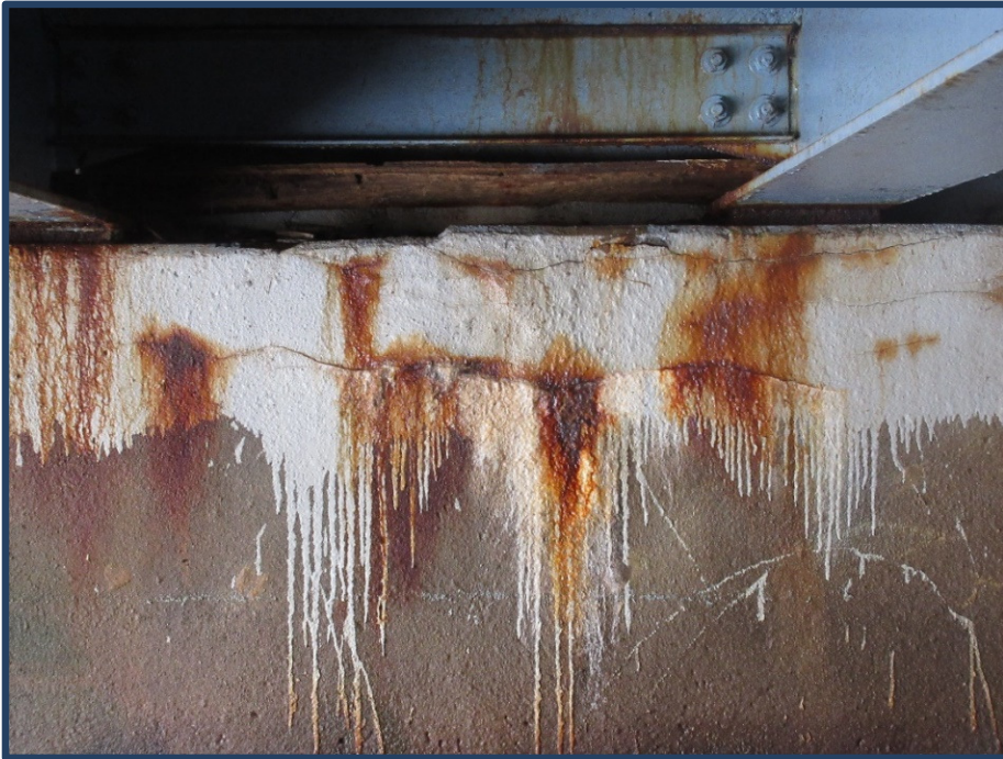
Abutment bearing seats
