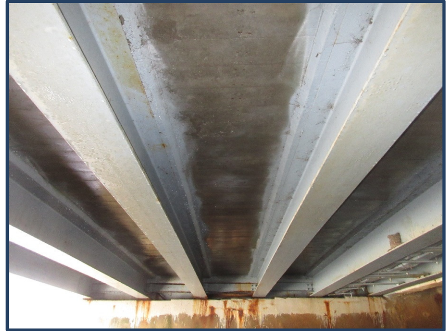
Under deck – Widened Section (1960)
