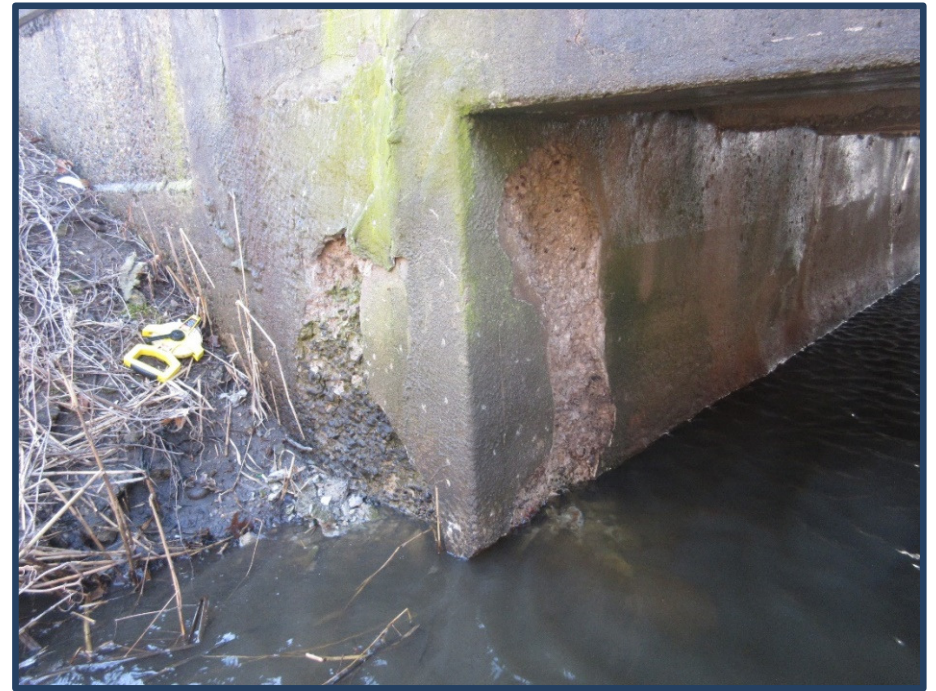
East Abutment - Northeast corner
