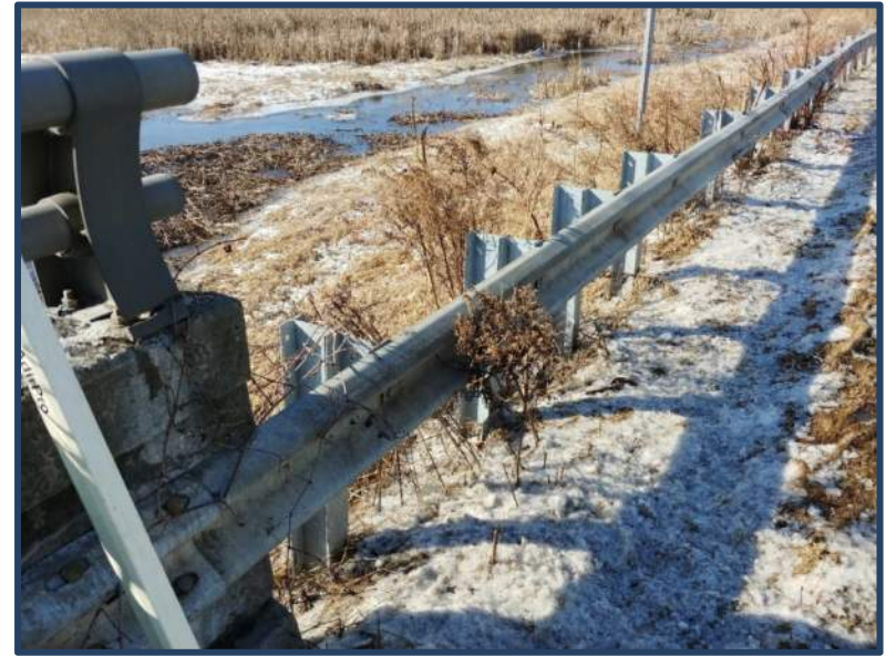
Substandard guiderail attachment
