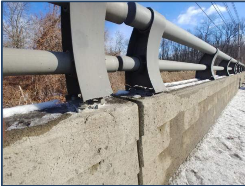
Damaged double rail element
